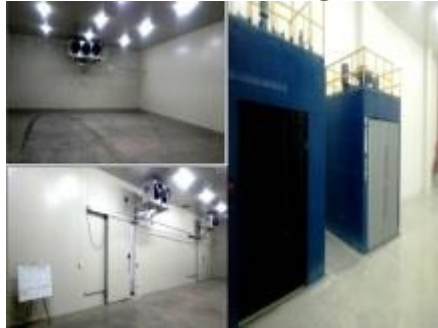
TCI's new cold chain warehouse
